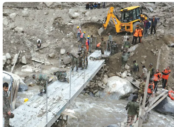
Figure 9.2: Army engineers working on a bailey bridge to restore connectivity to Chashoti.
