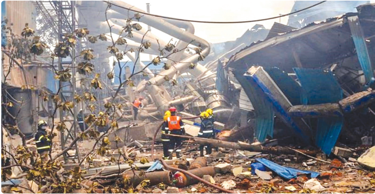
Figure 67: The extent of the explosion was such that entire portions of the factory collapsed.
