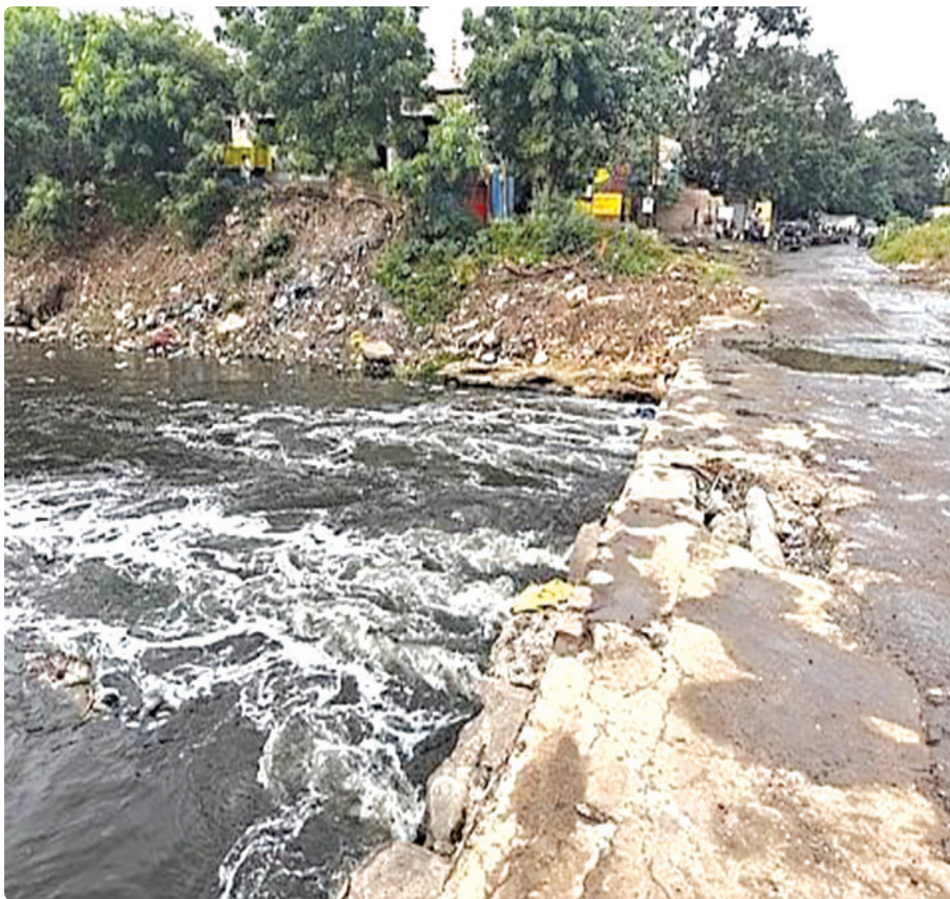
Figure 79: Sewage and solid waste flowing into the Kanh River in Indore near Goari Nagar bridge. Source: https://www.downtoearth.org.in/water/indores-clean-image-masks-a-liquid-waste-crisis
